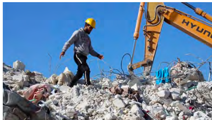
Rescue workers look for survivors amid the rubble of a building in the rebel-held town of Jindayris on February 9, 2023 (Photo: Mohammed AL-Rifai / AFP)
