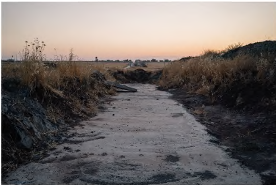
Syrian Kurdish officials say they have built concrete tunnels along the border, such as this one in the countryside of Hasakah, to prepare for a possible attack by the Turkish army. (Alice Martins for The Washington Post)
