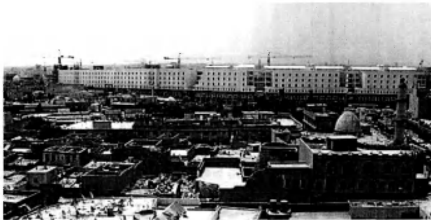
Construction cranes dot the skyline as a new shopping mall rises in Irbil.
