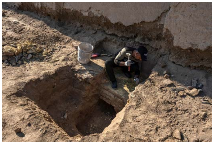
An Iraqi worker chiseling out modern concrete that was used in Babylon between the ancient brick and is now damaging it. Abdullah Dhiaa Al-deen for The New York Times
