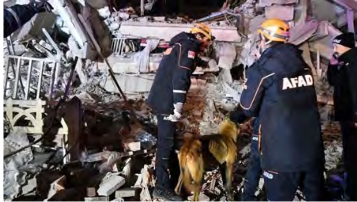
Rescue teams at the site of a collapsed building after Friday's 6.8 magnitude earthquake that shook mostly Kurdish-majority areas in southeast Turkey, Jan. 24, 2020. (Photo: AA)
