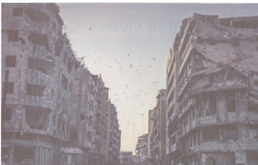
Destroyed apartment buildings in Homs, Syria, in 2014. Tens of thousands languish in Syrian government custody, where the conditions have been called a crime against humanity.
